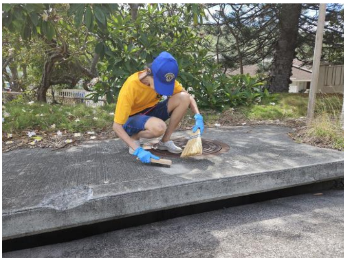
CIS Lyn Yee cleaning a section prior to placing storm drain marker.
