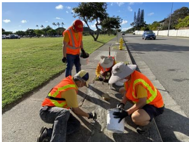
Hawaii Kai Lions repaving sidewalk with large crack dent.
